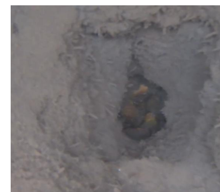
Accumulated mud on the gravel layer.
