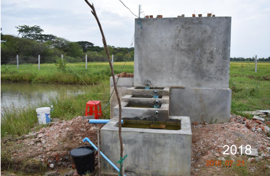
Mandalay, Myanmar: Pond → settling tank → 3 Up-flow Roughing Filters → Sand Filter → safe drinking water.
